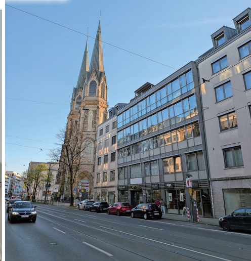
The building housing the representative office
